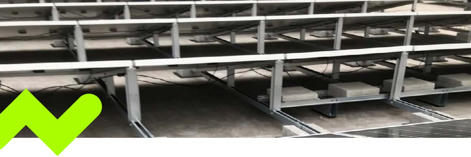
Align the rows according to plan, taking into account the width of the panels.
